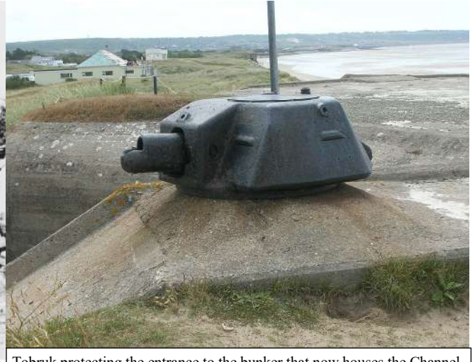
Tobruk protecting the entrance to the bunker that now houses the Channel Islands Military Museum. This turret was originally mounted on a Tobruk at Saint Aubin's Fort, Jersey.
