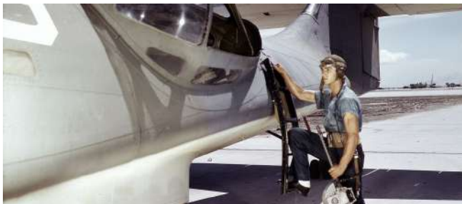
An Aviation Ordnanceman stationed at the Naval Air Station Corpus Christi installing an AN-M2 Browning machine gun in a PBY flying
