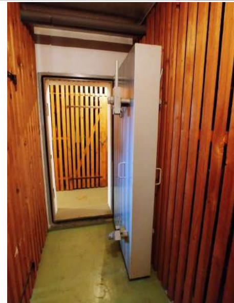
Switzerland cellar/Bomb shelter door. Until a few years ago every Swiss house had to have a bomb shelter, nowadays they are used as cellars.
